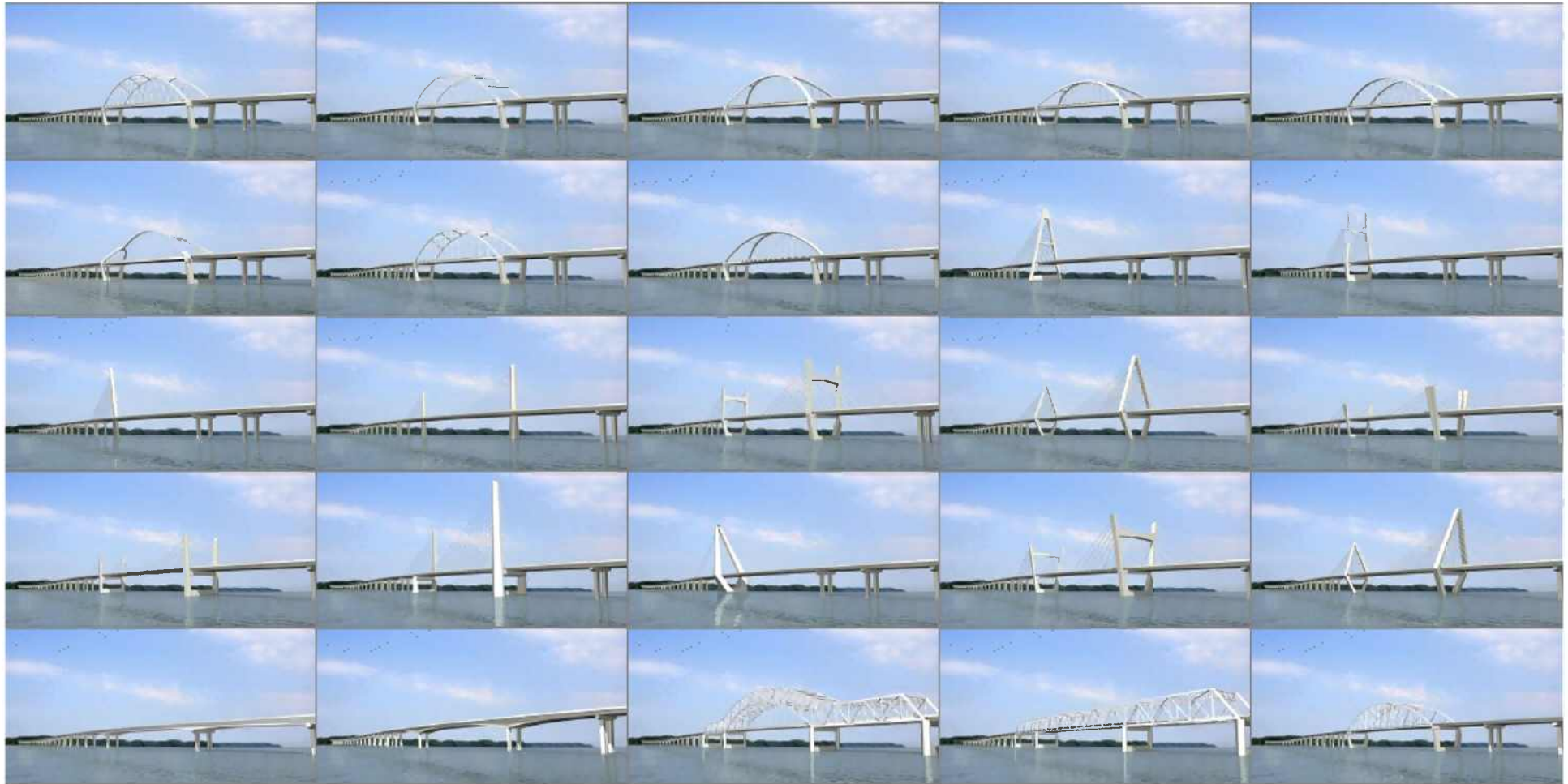
25 Bridge Concepts (8 Arches, 12 Cable Stays, 2 Girders and 3 Trusses)
